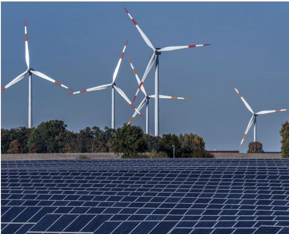
▲ Wind turbines turn behind a solar farm in Rapshagen (Germany)
