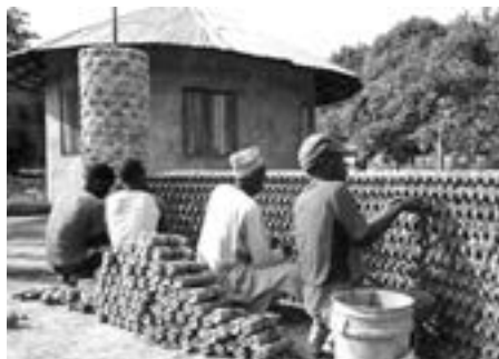
▲ The house is built of Ecobricks in Philippines
