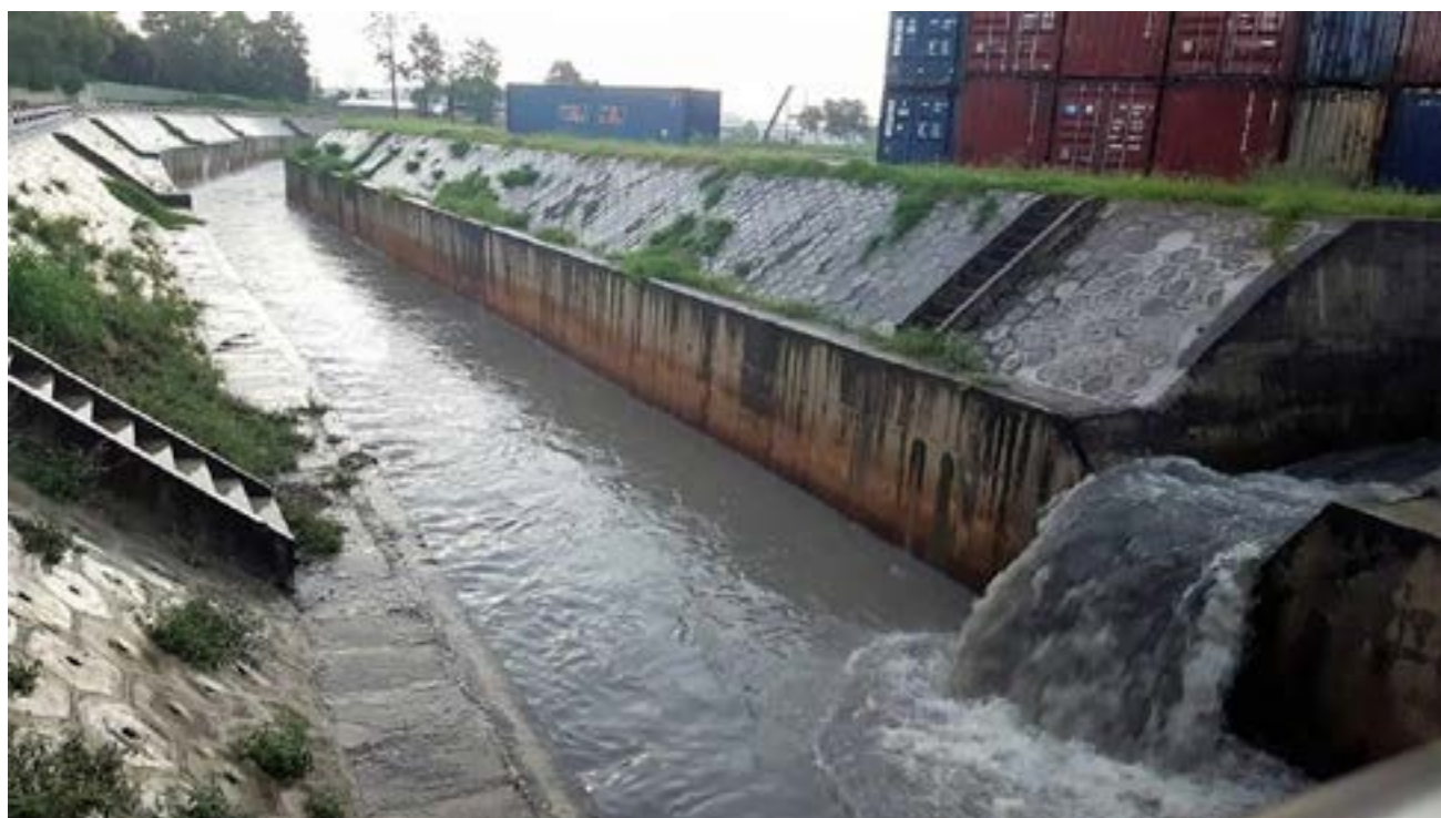
▲ The Ba Bò channel (the section passing through Bình Dương province) was dredged, cleaned, renovated and embanked
