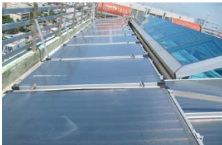
▲ Solar panels on the roof of a residential apartment in Đà Nẵng, 30% of the city's population are using solar powered water-heaters.
