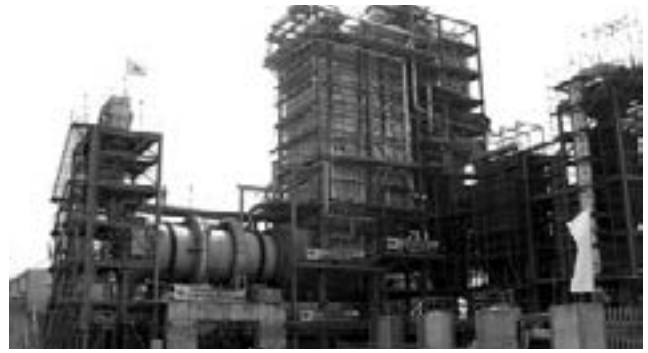
▲ The first waste energy system in Việt Nam
